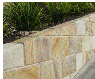
ST STONE CLADDING SANDSTONE CLADDING TO GROUND FLOOR PERIMETER WALL & PLANTER BOX
