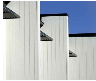
RW2 RENDERED WALL - TYPE 2 Rendered wall with groove lines Colour - (P3) Dulux- Paramount Design (SN4E2)
