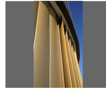
ALP ANODISED ALUMINIUM PROFILE SATIN QUARRY BEIGE FROM UNIVERSAL ANODISERS or similar
