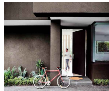
RW RENDERED WALL Colour - (P1) Dulux- Brown Fox (P11A8) Colour - (P2) Dulux- Caps (PN2B5) Colour - (P5) Dulux - Kahlua Milk (P15C3)
